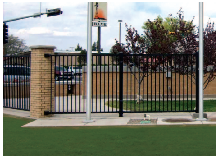
STRONGRAIL® outlines the entrance to the New Mexico Military Institute. The fiberglass fencing's low maintenance, ease of installation and aesthetic quality were driving factors behind the institute's selection of STRONGRAIL®.
