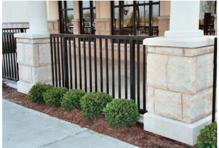
A custom handrail system installed for Karlo's Bistro blends with surrounding architecture and adds aesthetic appeal.
