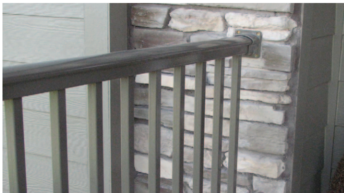
STRONGRAIL® with square pickets and a rounded top rail was produced in a custom color to compliment the exterior of this residential area.
