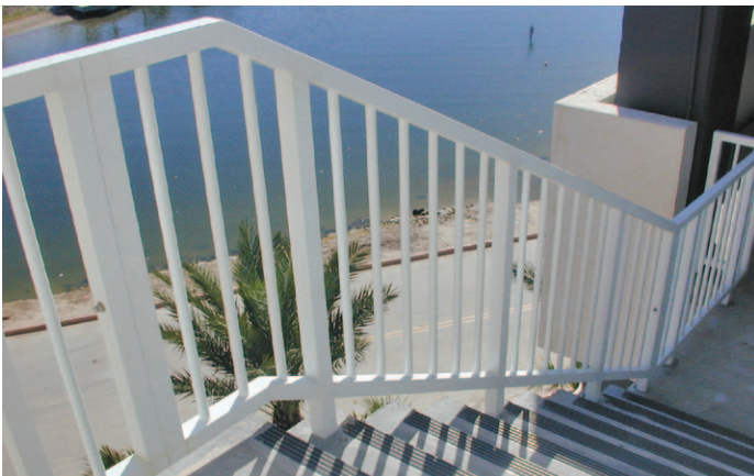
The Moody Gardens Convention Center parking garage in Galveston, Texas is also outfitted with STRONGRAIL®. The durable fiberglass architectural handrail system is the ideal solution for a building that experiences high levels of traffic like this one.
